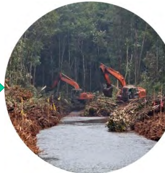
Canals built to drain water
