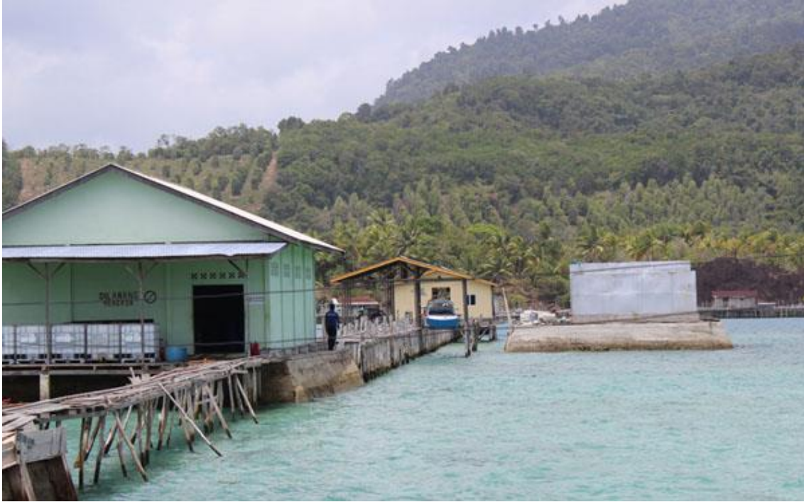
Figure II-18. The only one fuel station at Anambas Archipelago owned by Mr. Akin
