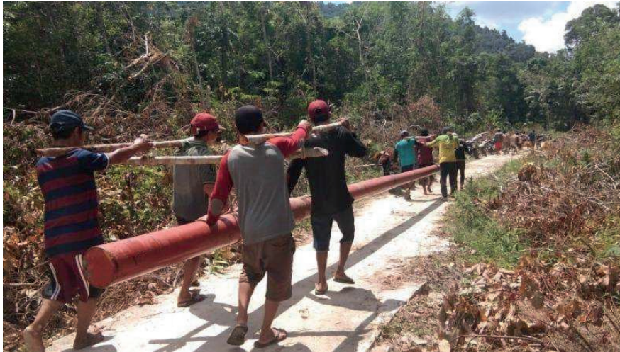
Figure 1.2 Residents of a village on the island of Kalimantan work together carrying electric poles as part of a village electrification project (photo: ecuator.co.id, 2019).
