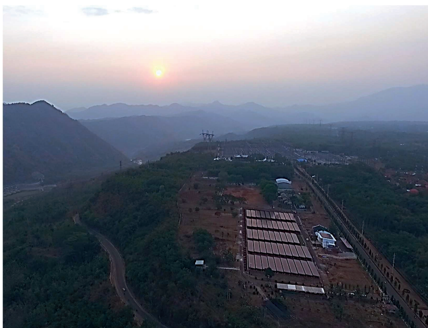
Figure 6.1 Aerial view of the 1 MWp PV plant in Cirata, West Java, Indonesia (Photo: PJB Cirata).
