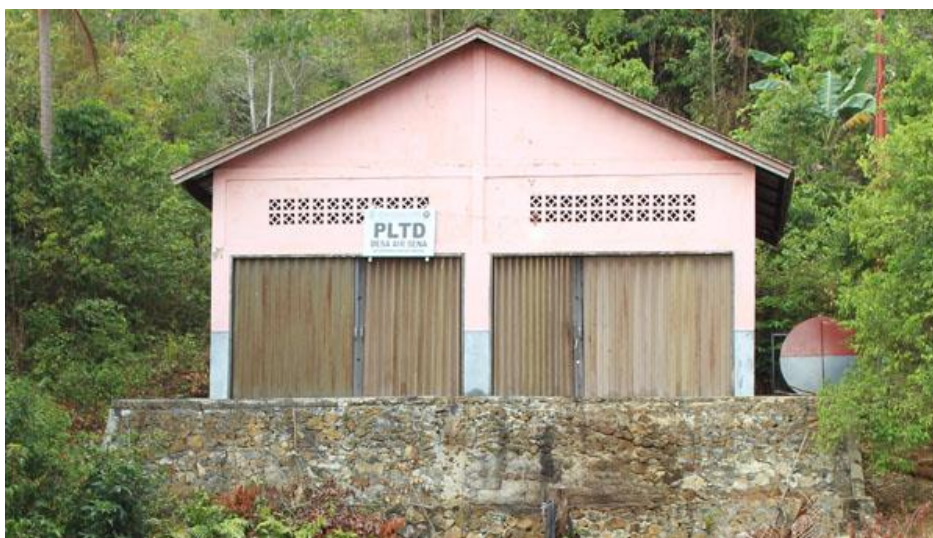
Figure III-1. The front view of the Diesel Power Plant
