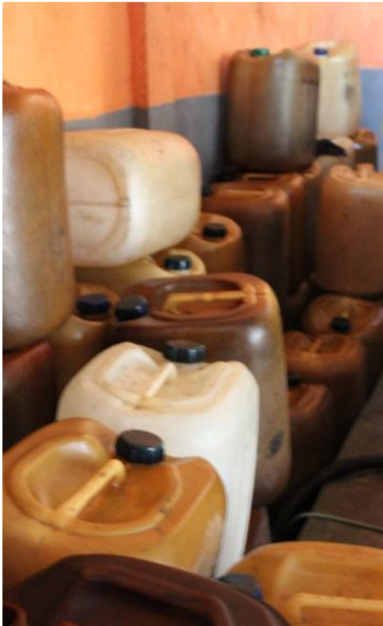
Figure III-4. Gallons used for fuel storage at the PLTD Air Sena Village
